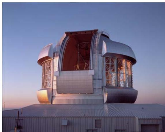
Gemini North dome/enclosure with setting sun (to left) lighting up the bottom half of the telescope through thermal vents (fully open). The observing slit is partially open, revealing the truss and top end of the telescope. *Credit: Neelon Crawford - Polar Fine Arts; courtesy of Gemini Observatory and NSF*
