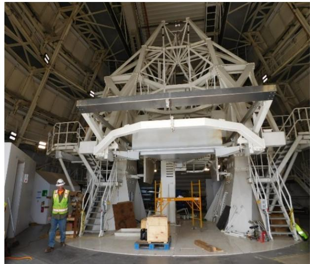
The Telescope Mount as of July 2017, showing two recently-completed Nasmyth platforms left and right of the main structure. Credit: P. Jeffers NSO/DKIST.
