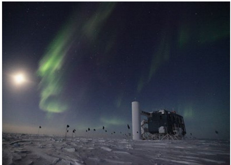
The IceCube Laboratory building at South Pole where all data-collecting computer servers are located. Credit: USAP Photo Library, Sven Lidstrom, NSF.
