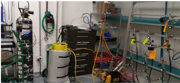
Installation and flushing of the refrigeration lines (Oct 2019)
