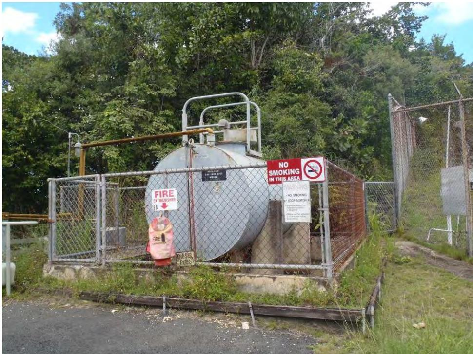
*Photo 54: 2,000-gallon diesel tank for emergency generator facing west.*
