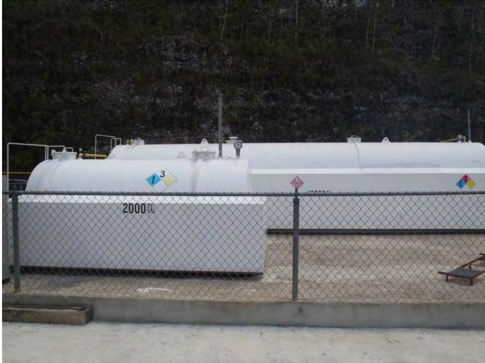
*Photo 53: 2,000-gallon gasoline aboveground storage tank and 12,000-gallon diesel aboveground storage tank facing south.*
