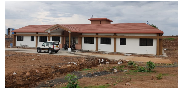
Site office at the LAO site
