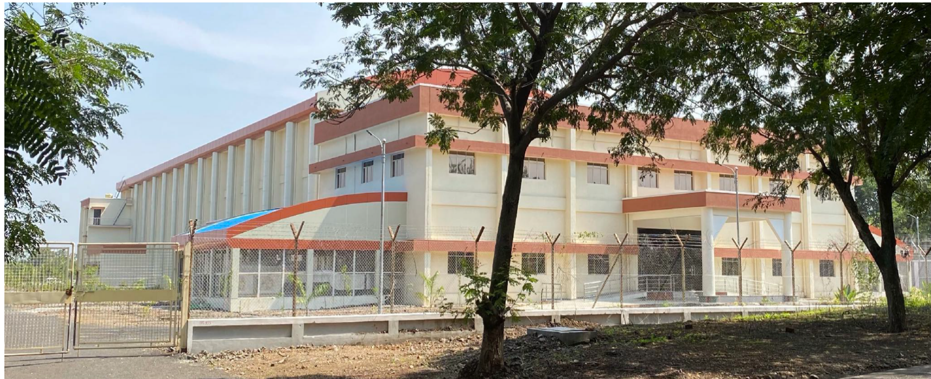
Staging and testing facility & 3G R&D
