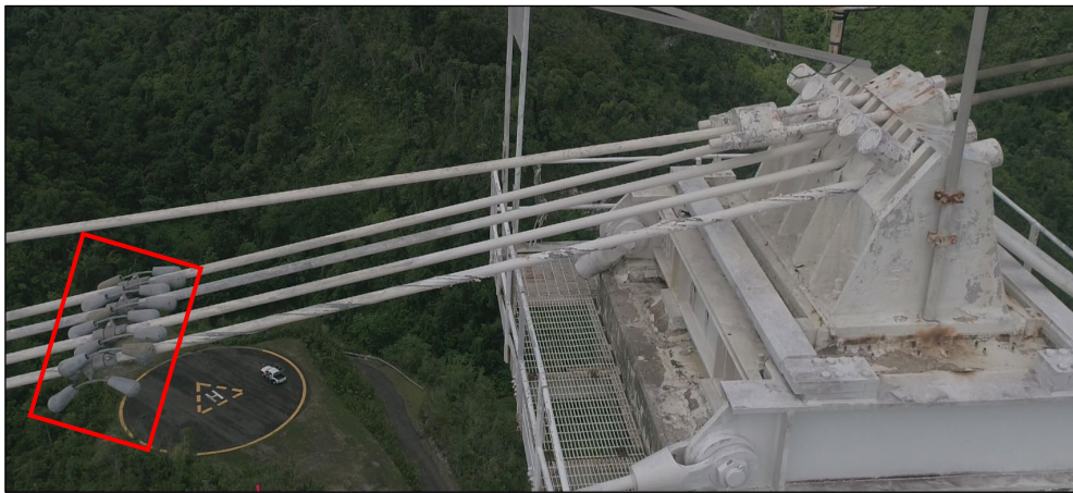
Figure 7: Stockbridge dampers on Tower 4 original mains.
