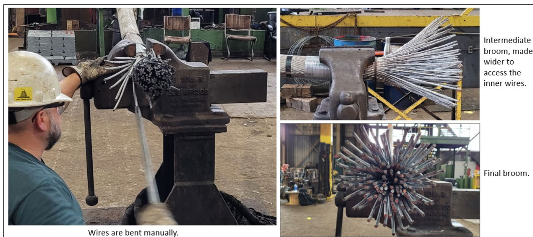
Figure 3: Manual wire brooming.
