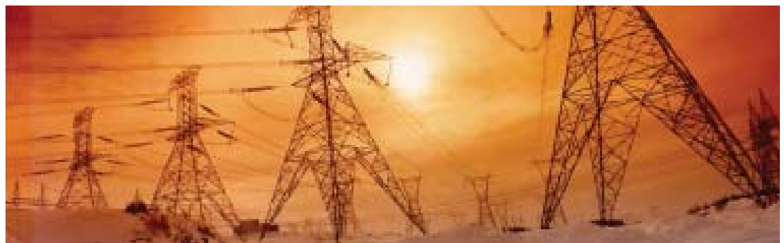
735 kV transmission lines.
