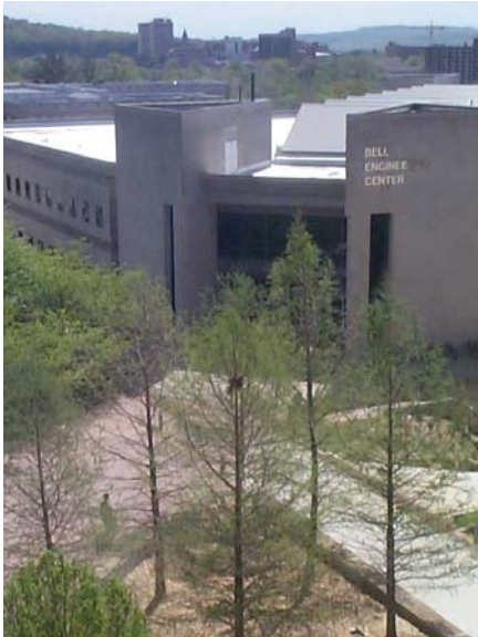
Bell Engineering Center, University of Arkansas
