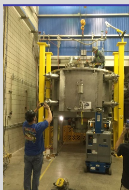
Figure 1. The Series-Connected Hybrid (SCH) magnet during installation.
