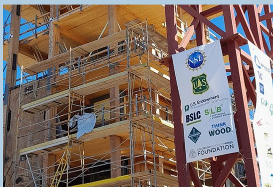
The 10-story mass timber building under construction on the shake table. Credit: Shiling Pei/Colorado School of Mines.
